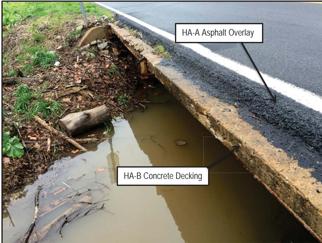
Photo 1: View of HA-A and HA-B on the top of SR-223 Bridge over Branch
