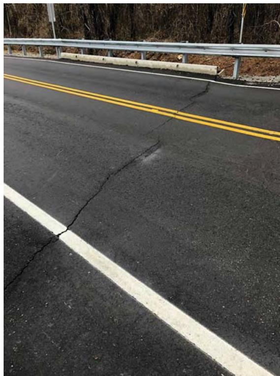
Pavement Cracking at East Abutment Connection
